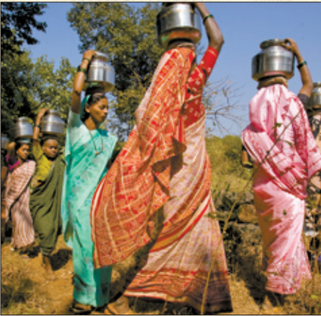
Together with SHARE, Rotarians and village volunteers built a retaining wall to keep wells from going dry in Mandatane, India.
